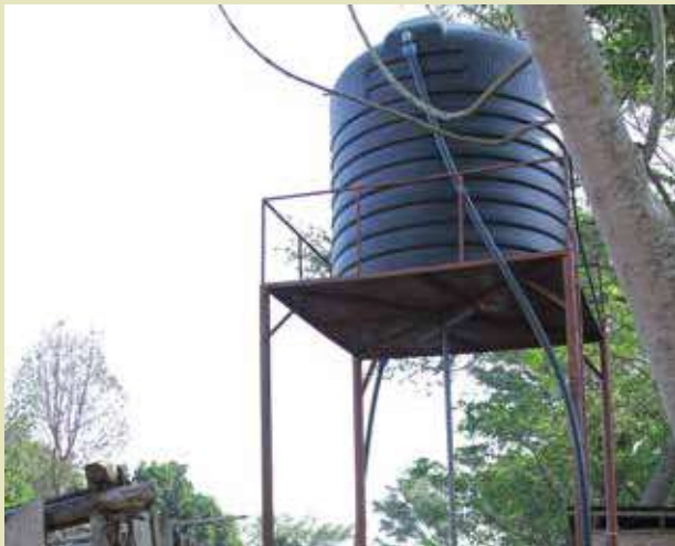
Overhead water reservoir
