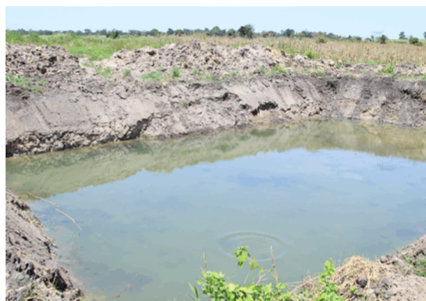
Figure 18: Water harvesting dam for providing water to a mother garden
