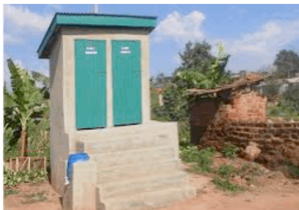
Figure 3: A pit latrine facility at a clonal Coffee nursery
